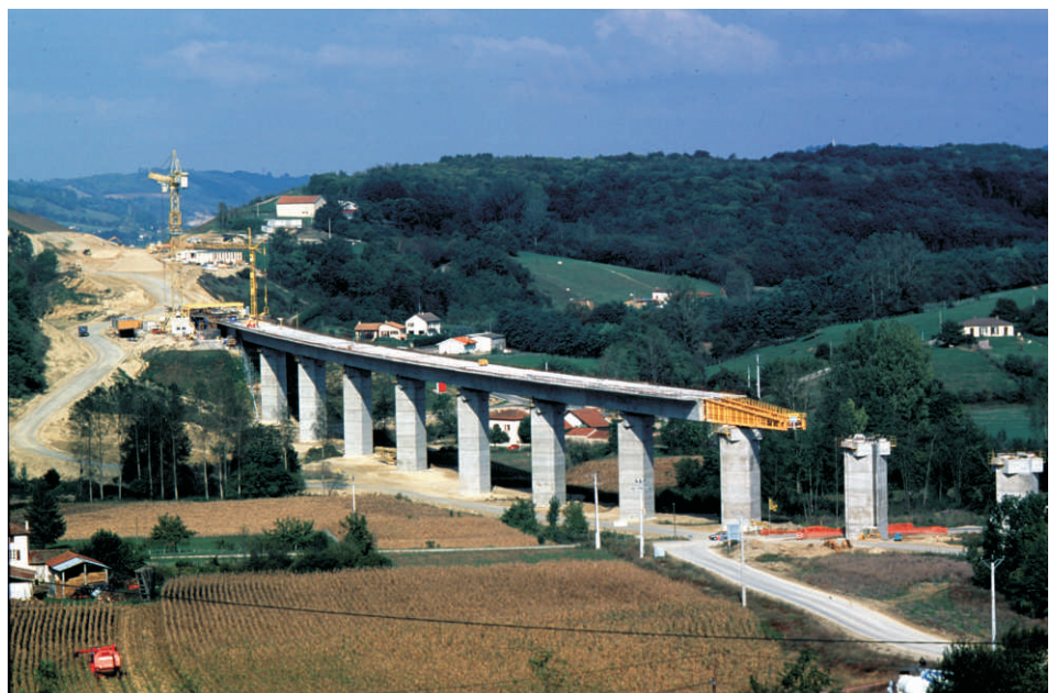
Meyssiez TGV Viaduct: general view
