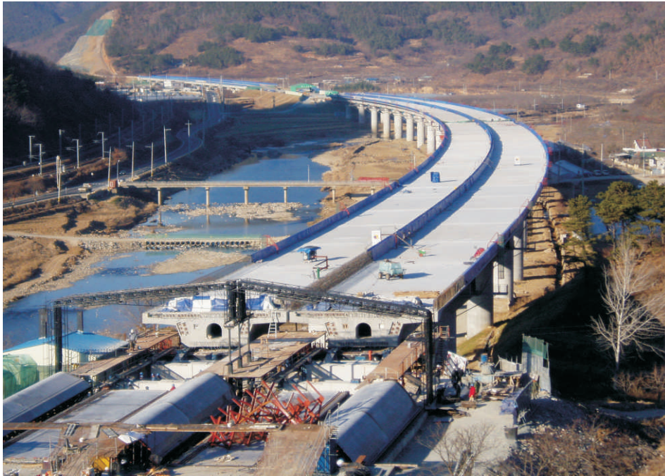
Dansan Bridge construction
