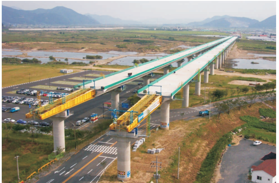
Miryang Grand Bridge, Korea
