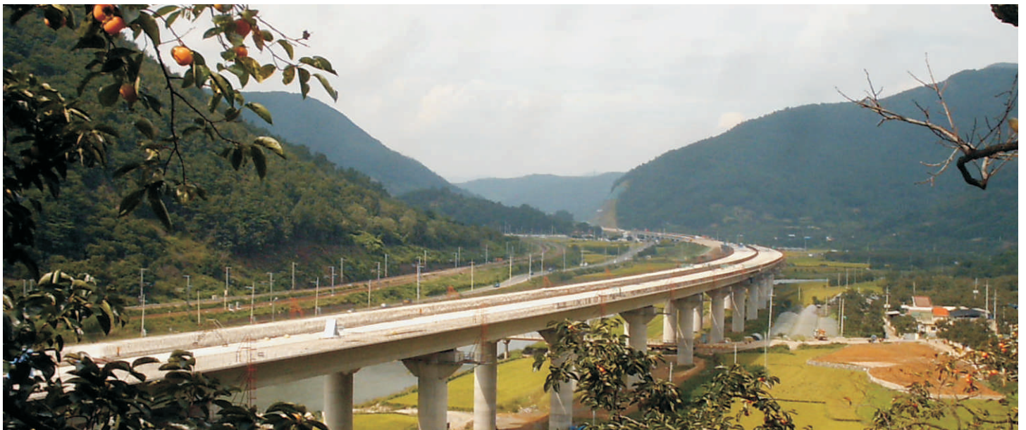
Dansan Bridge, Korea
