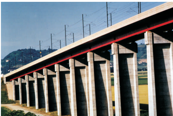
Meysiesz Viaduct, France
